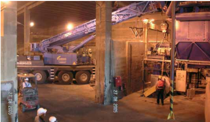
Austausch des Zerkleinerungsaggregats / Exchange of the shredder aggregate
